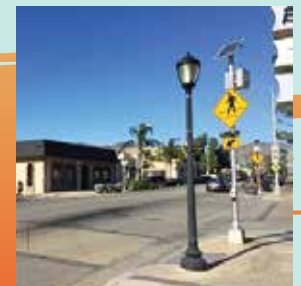
Street and crosswalk lighting
