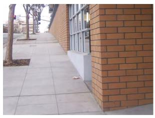
Brick veneer wraps the corner and is detailed to look like load bearing masonry.
