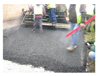
Figure 9: Permeable Asphalt Installation Using Ground Tire Rubber.
