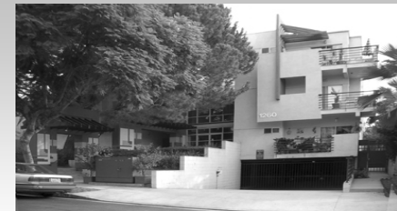
Transition to the yard and support for the balconies above are missing from this ramp.
