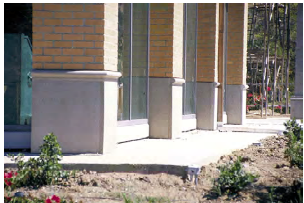
A building base can be created by a visibly thicker portion of the wall along the ground.
