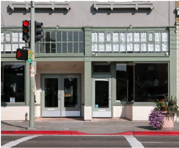
Storefront bases can be made of precast or poured-in-place concrete.
