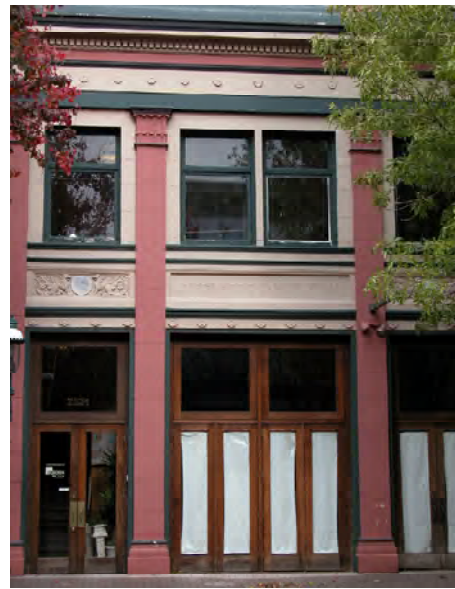
Flat roofs should be edged with architecturally profiled cornices,
