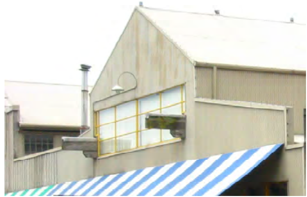
Corrugated and standing-seam metal roofings should be carefully detailed so that roof edges will not sag or bend.
