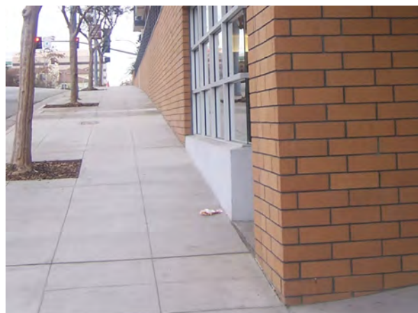
Brick veneer wraps the corner and is detailed to look like load bearing masonry.
