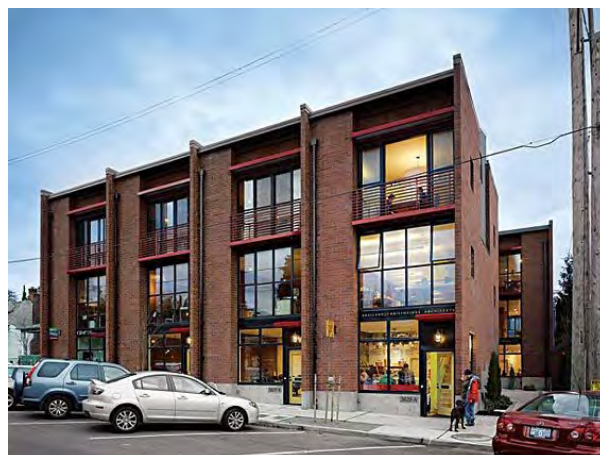
A 3-story live-work building clad in brick over a cast-in-place concrete base.
