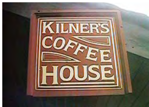
Wood is a recommended material, as shown on this sign with incised letters cut into a wood sign panel.
