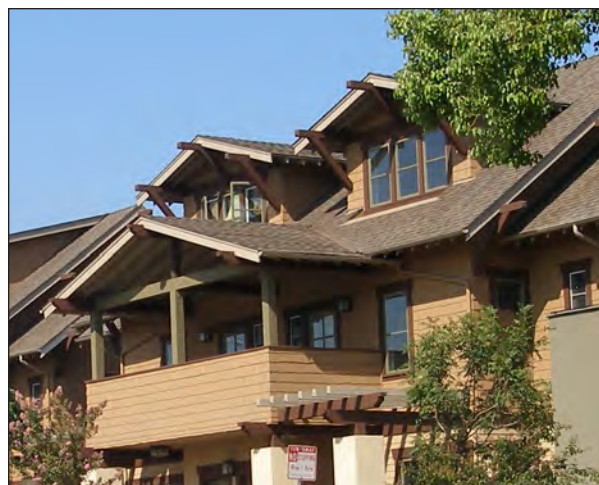
Upper floors are incorporated into the attic spaces and are daylit by dormer windows.
