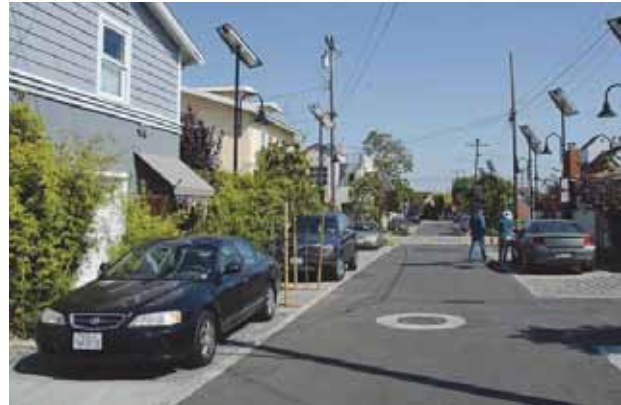
This street has removed curbs and uses textured pavement to visually narrow the street and invites people to walk down the middle.
