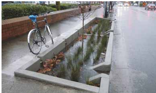
Curb cut-outs in depressed tree well/parkway allow water to seep in, be stored, and cleaned through system
