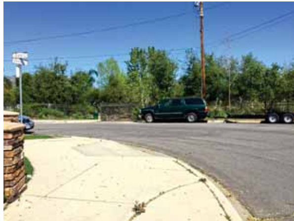
Ramp missing truncated domes for visually impaired users at Eighth Street and Newton Street
