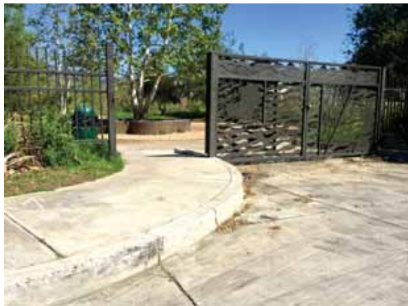
Missing curb ramp and truncated domes at entrance of Pacoima Wash Natural Park
