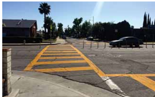
Uncontrolled marked crossing of Glenoaks Boulevard at Alexander Avenue with Rectangular Rapid Flashing Beacons. Plastic pylons prevent vehicular crossings of Glenoaks Boulevard. The crossing distance is approximately 75' from the edge of each ramp.
