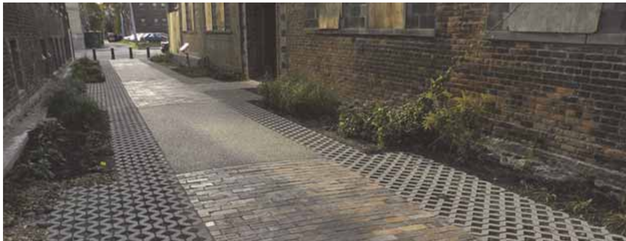
Green Alley uses bricks and permeable pavers to create a more inviting walking space and recapture water
