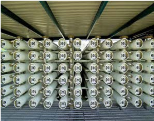
Reverse Osmosis Membranes at West Basin Municipal Water District, Brewer Desalination Facility. Desalination of local brackish groundwater helps reduce the Region’s dependence on imported water.
