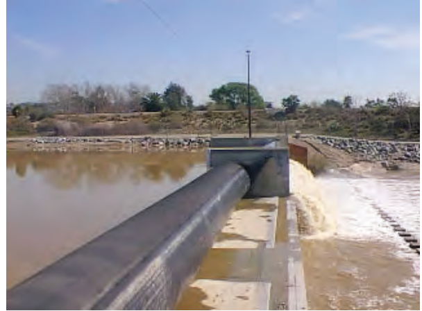
LACFCD operates inflatable dams on the San Gabriel River to promote short-term in stream recharge.
