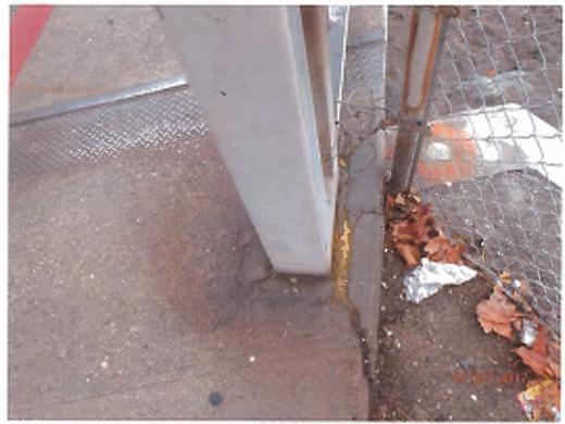
Photo 5 - Spalling Rail End
