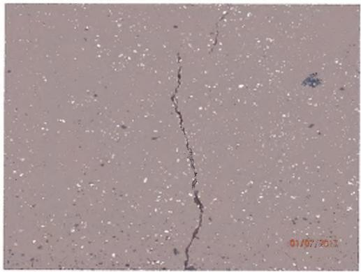
Photo 3 - Deck Cracking Example
