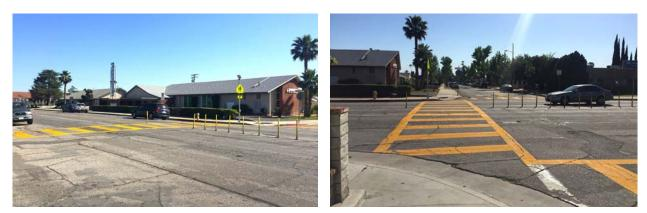
Uncontrolled marked crossing of Glenoaks Boulevard at Alexander Avenue with Rectangular Rapid Flashing Beacons. Plastic pylons prevent vehicular crossings of Glenoaks Boulevard. The crossing distance is approximately 75' from the edge of each ramp.
