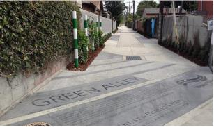
Green Alley built by Trust for Public Land in collaboration with City of Los Angeles that uses permeable surfaces to cool temperatures and collect water
