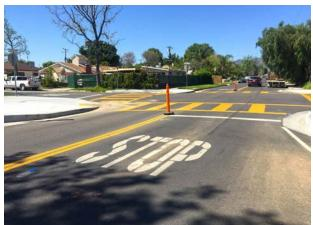
Advanced stop bars (bar behind crosswalk, in front of STOP pavement legend) show drivers where to stop, and help prevent cars from encroaching into the crosswalk. San Fernando has installed curb extensions and upgraded pavement markings throughout the city
