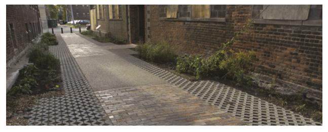
Green Alley uses bricks and permeable pavers to create a more inviting walking space and recapture water
