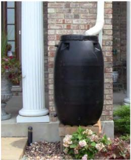
Figure 7.10: Rain Barrel
