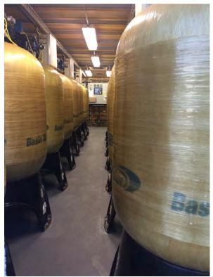
Figure 2.9: Ion-Exchange Facility at Well No. 7A
