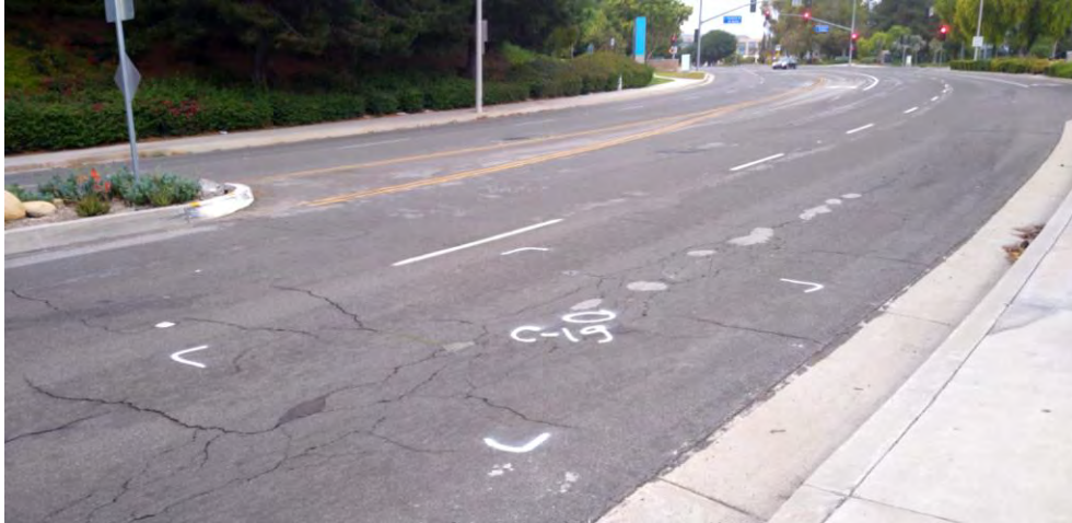
Photo 5: Coring location C-19 on Enterprise in Aliso Viejo. Pavement contains alligator cracking, depression, and potholes.
