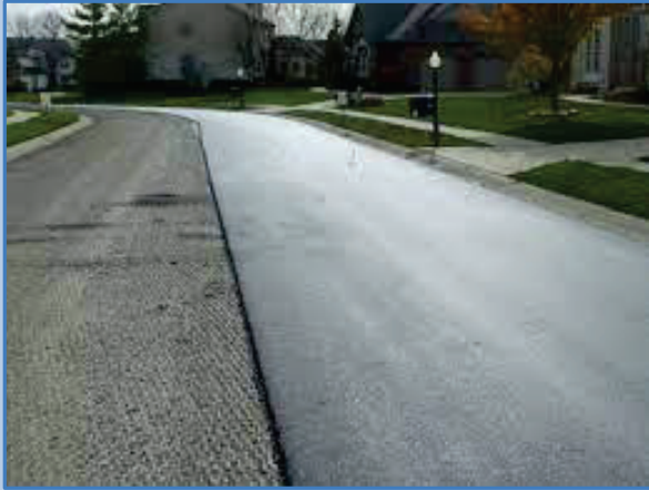
Thin Asphalt Overlay
