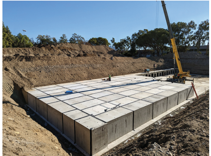
THE CITY CONSTRUCTED A NEW WATER INFILTRATION SYSTEM
