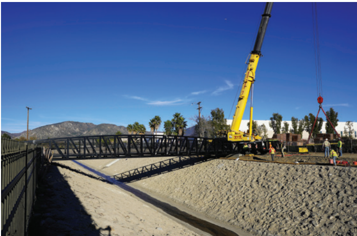
PACOIMA WASH BIKE PATH BRIDGE INSTALL
