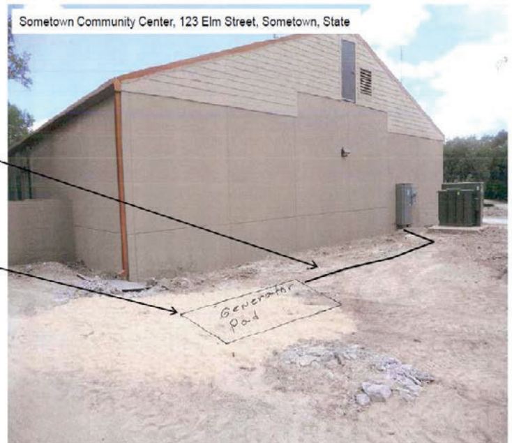
Figure 4. Ground-level photograph showing proposed ground disturbance area.
