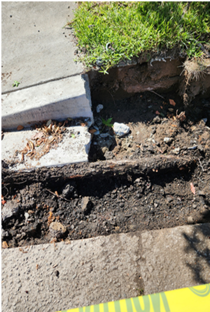
454 Kalisher Street - Root under gutter. Root pruning will cause tree to be unstable. Root invasion was not visible during initial walk-thru of job site. No proposed replacement – Water meter and driveway approach within close proximity. Parkway has 4 existing trees
