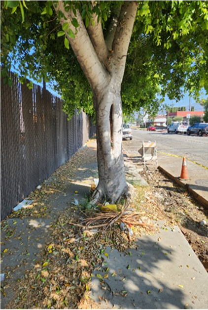
1115 First Street – Roots under gutter. Root pruning will cause leaning tree to be unstable. Root invasion was not visible during initial walk-thru of job site. Replacement Options: Carrotwood, Long Leafed Yellow-wood
