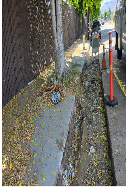
1115 First Street – Roots under gutter. Root pruning will cause leaning tree to be unstable. Root invasion was not visible during initial walk-thru of job site. Replacement Options: Carrotwood, Long Leafed Yellow-wood
