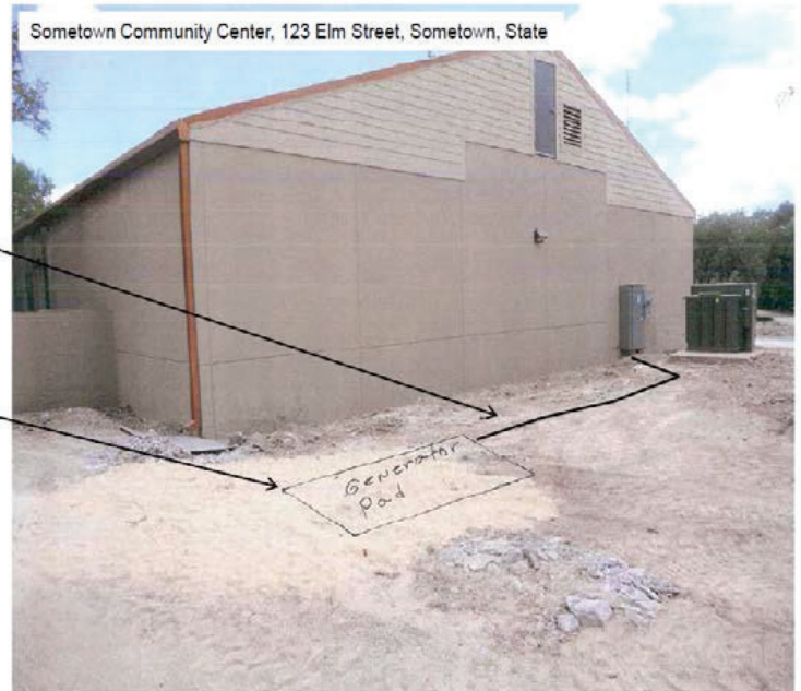
Figure 4. Ground-level photograph showing proposed ground disturbance area.
