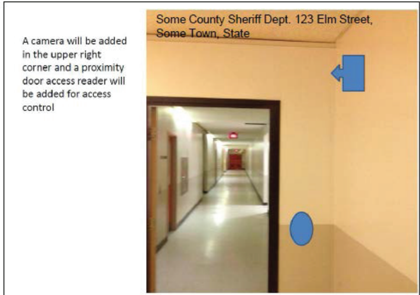
Figure 6. Interior photograph showing proposed location of new equipment.
