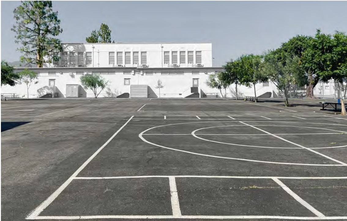
Image 27. The schoolyard consists mostly of asphalt with a small, poorly maintained lawn. Lack of shade can result in ambient temperatures over 142 degrees Fahrenheit (Green Schoolyards Plan - Los Angeles 2024)
