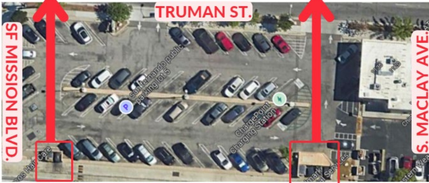
ALLEY 1 | PUBLIC PARKING LOT 5
