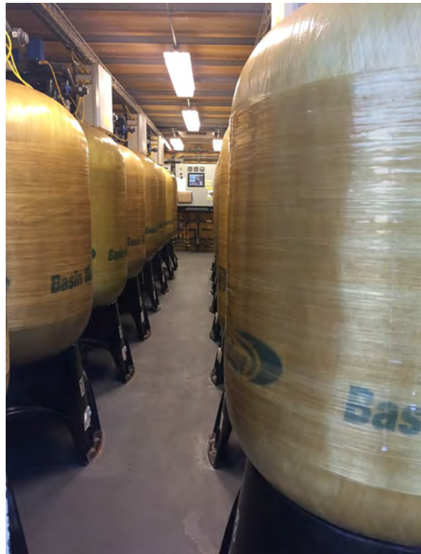
Figure 2.9: Ion-Exchange Facility at Well No. 7A
